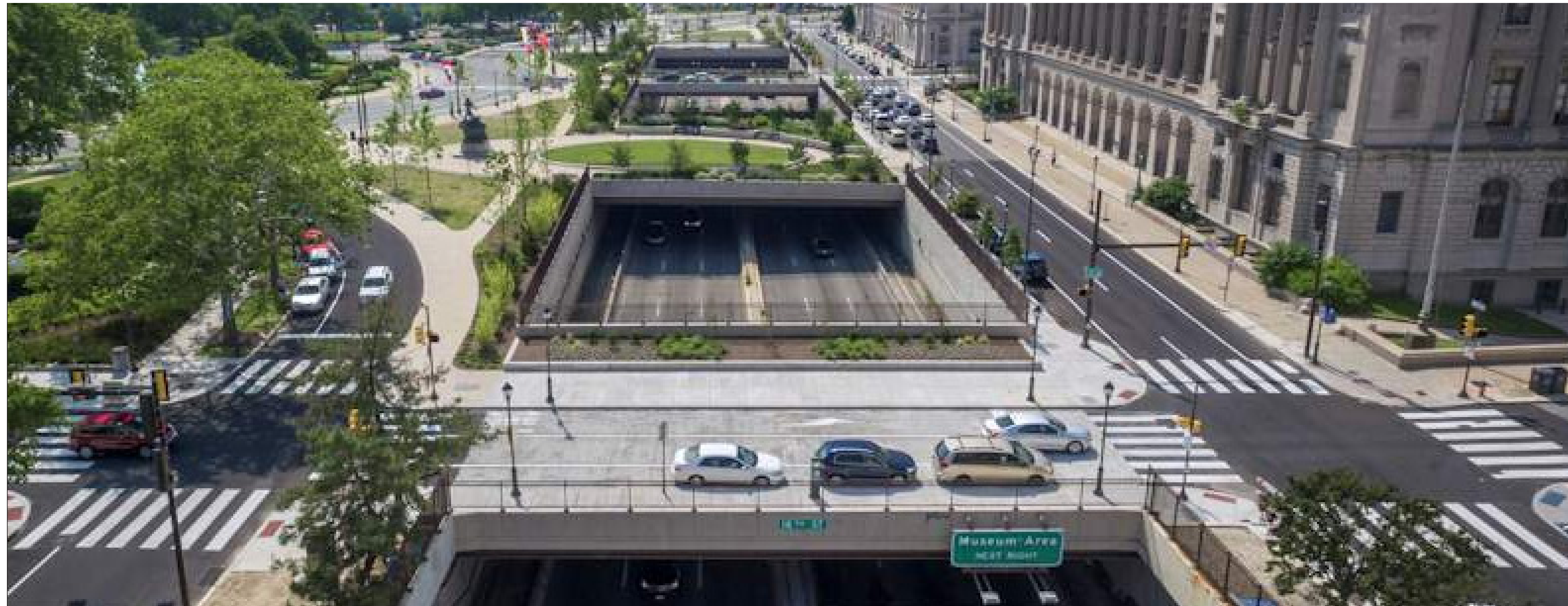
Vine Street Expressway, Philadelphia, partial highway cap
